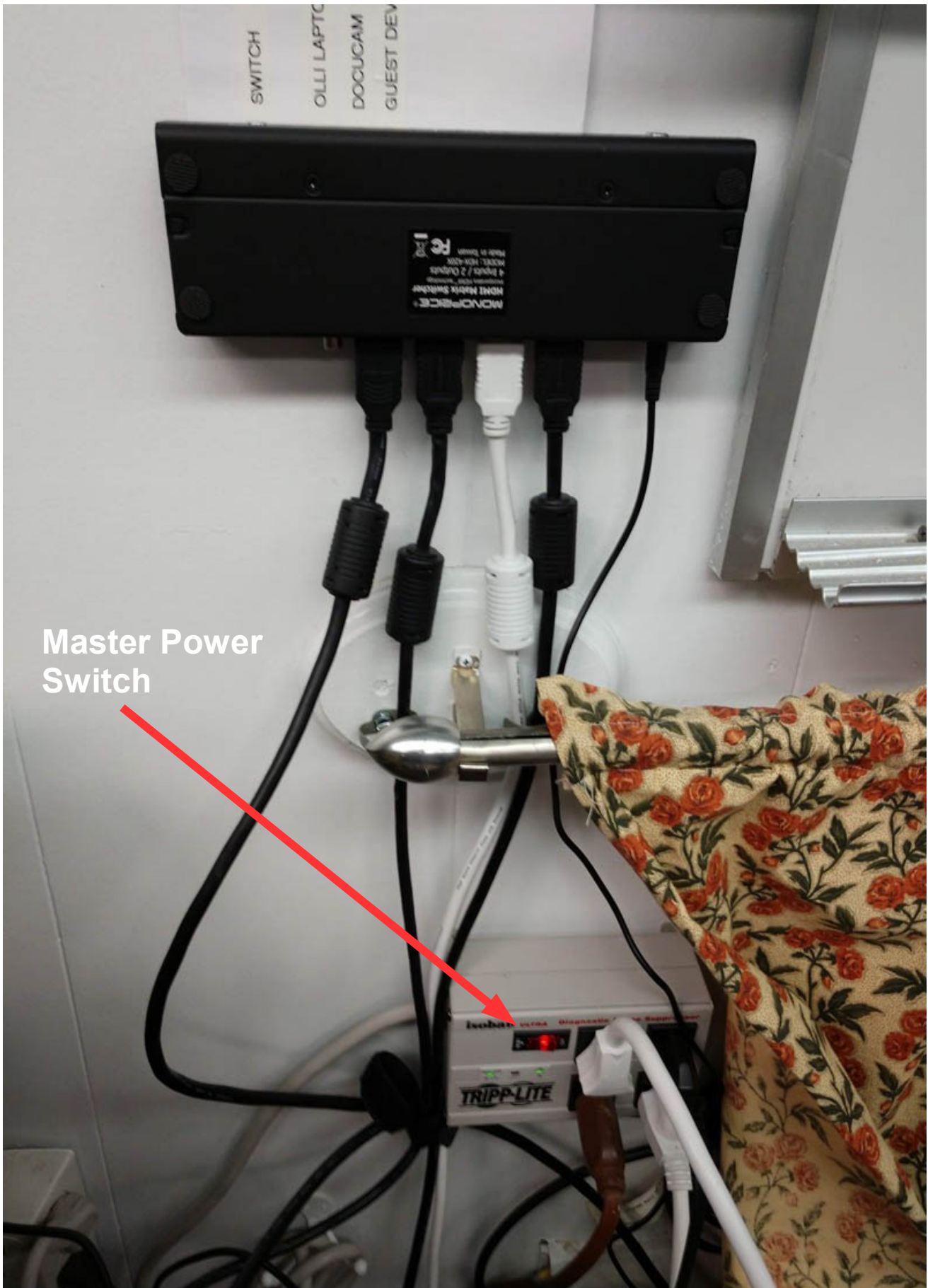
TA1 Master Power switch for podium area electronics – laptop, docucam, guest power strip.
